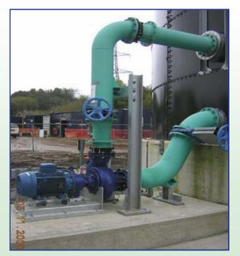
Traditional method of mixing anaerobic sludge digesters
